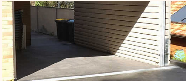
Rainwater tanks incorporated into a carport design shows clever and effective use of small spaces
