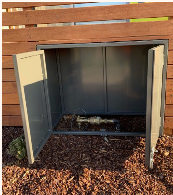
Integrated water meter details within courtyard walls
