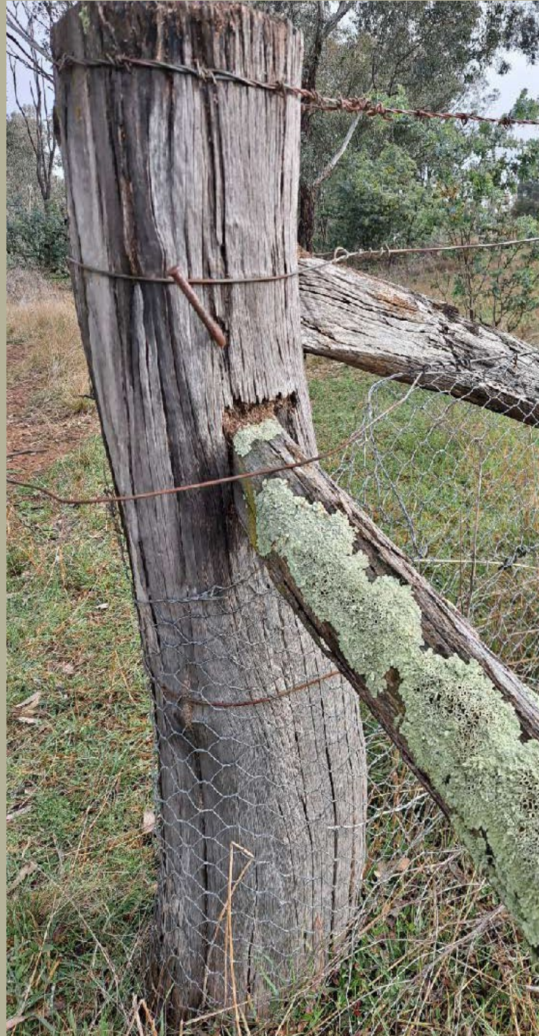
Figure 31. Original timber fence posts within the Conservation Corridor
