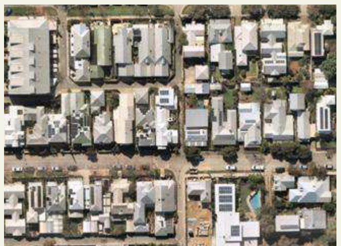
Lighter roofs reduce heat transfer
