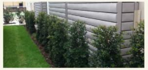
Narrow style rainwatrer tanks can be used where space requirements are restrictive
