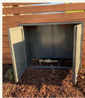
Integrated water meter details within courtyard walls
