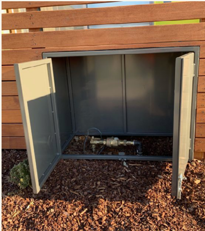
Integrated water meter details within courtyard walls
