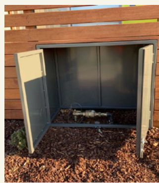
Integrated water meter details within courtyard walls
