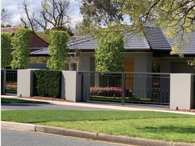
Open form powder coated metal gates and rendered masonry piers.
