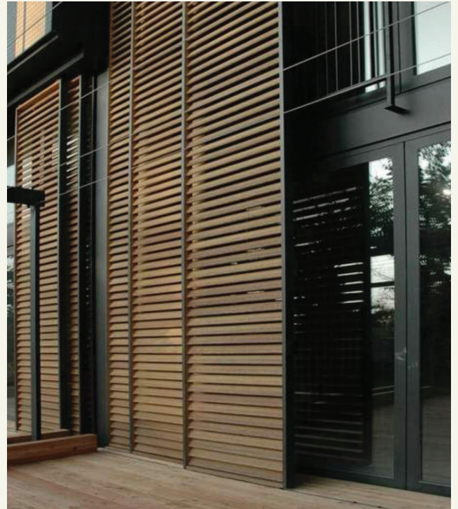
External screens to shade western façades.
