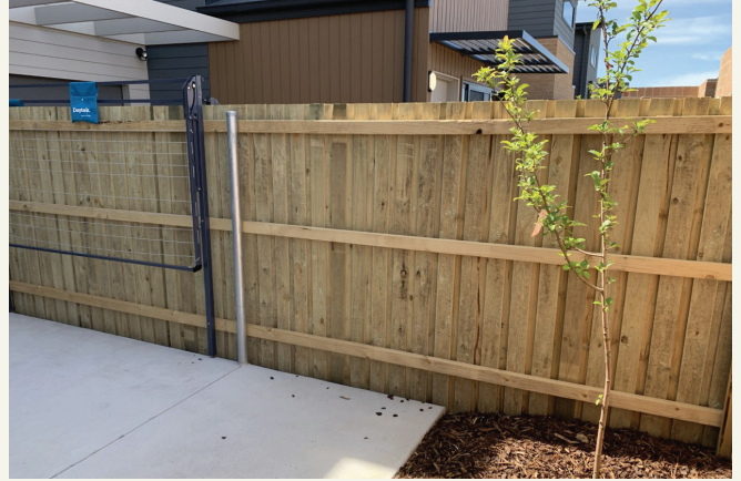
Timber inter-allotment fencing.
