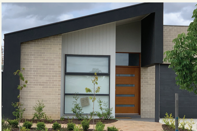
Integrated roof line and single post provides a well covered and visible entry.
