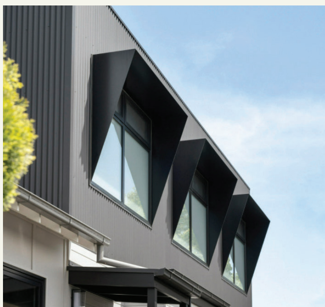
Awnings provide weather protection and permit better operability of windows and cross ventilation.
