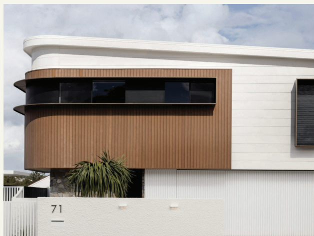
Example showing sunhoods to windows.
