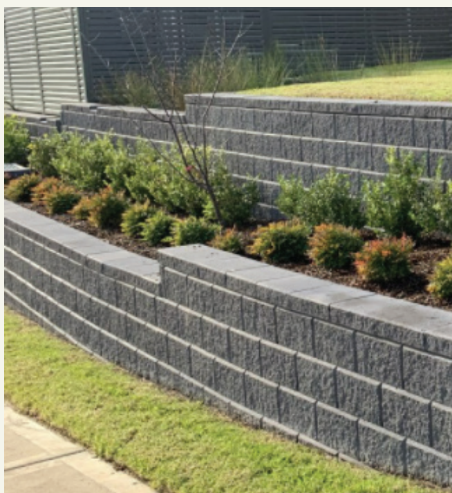
Architectural split face block with capping stone terraced to reduce a single wall height.
