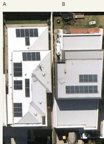
Example A: Hip roof design with complicated solar panel configuration
