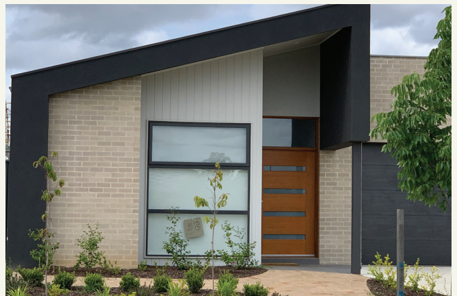
Integrated roof line and single post provides a well covered and visible entry.
