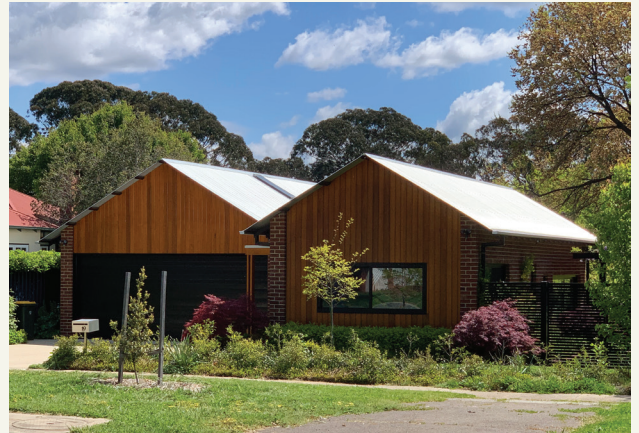
Example of a stained timber façade
