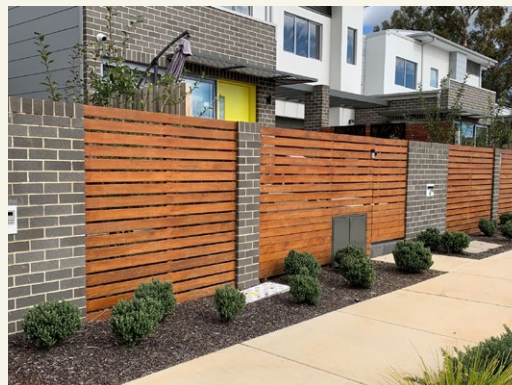
Clear entries behind courtyard walls
