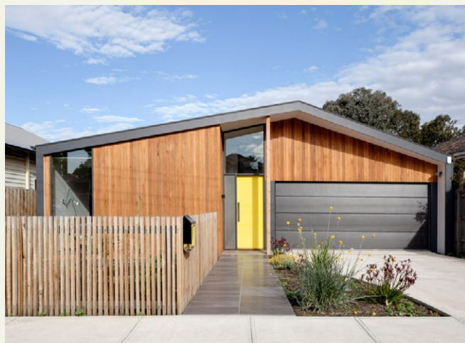
Example of panel lift doors showing stained hardwood cladding and vertical glazed elements
