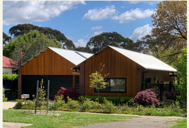
Example of a stained timber façade
