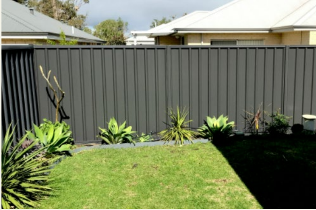
Side and rear fencing establish the inter-allotment boundaries. Ginninderry permits either “Jasper” colorbond or timber fencing.
