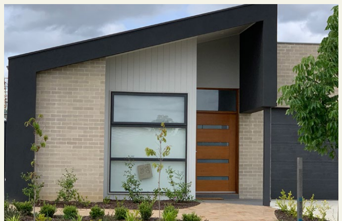
Integrated roof line and single post provides a well covered and visible entry.
