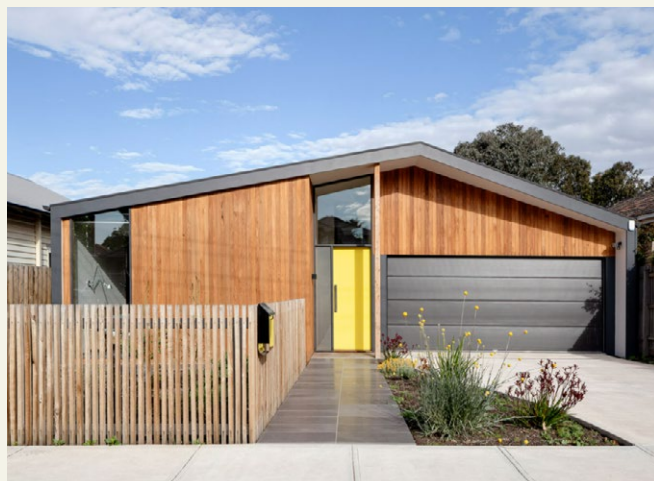
Example of panel lift doors showing stained hardwood cladding and vertical glazed elements
