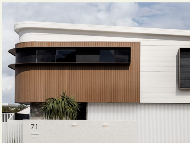
Example showing sunhoods to windows.
