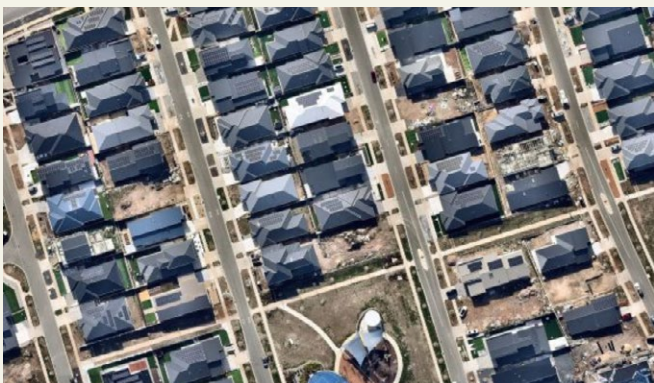
Darker roofs create excessive heat
