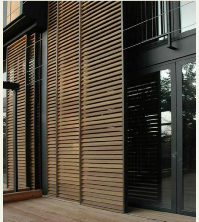
External screens to shade western façades.
