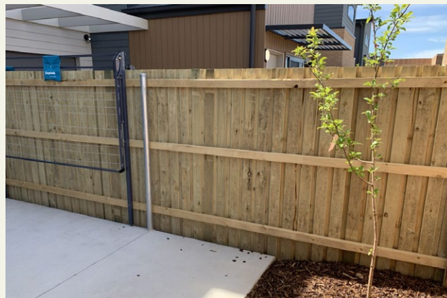
Timber inter-allotment fencing.
