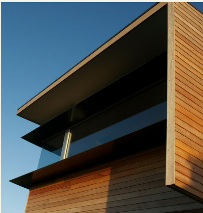
Window hoods and strong eave lines can inform the Architectural form whilst providing efficient shading and weather protection.
