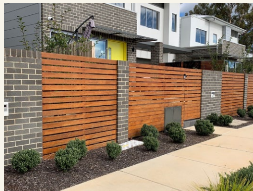
Clear entries behind courtyard walls
