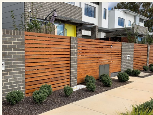
Clear entries behind courtyard walls
