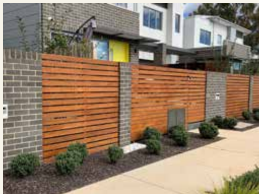
Clear entries behind courtyard walls
