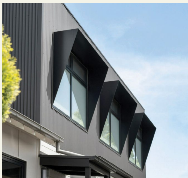
Awnings provide weather protection and permit better operability of windows and cross ventilation.
