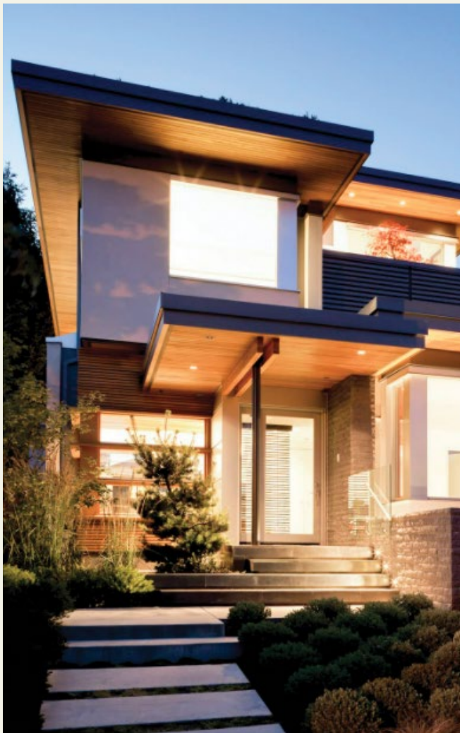
A post and beam supporting a partial cantilever style porch entry is open and welcoming from the streetscape.
