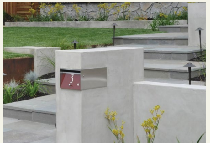
Mailbox integrated into a rendered pier and retaining wall.
