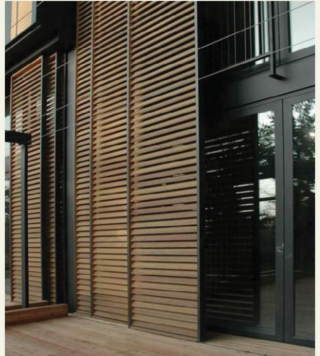
External screens to shade western façades.
