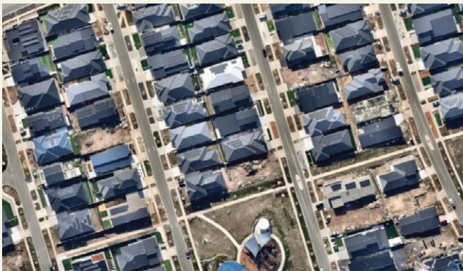
Darker roofs create excessive heat
