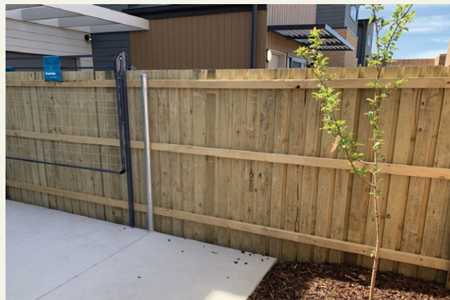
Timber inter-allotment fencing.
