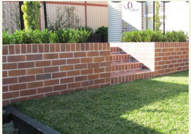
Smooth face brick retaining wall with accent planting behind.
