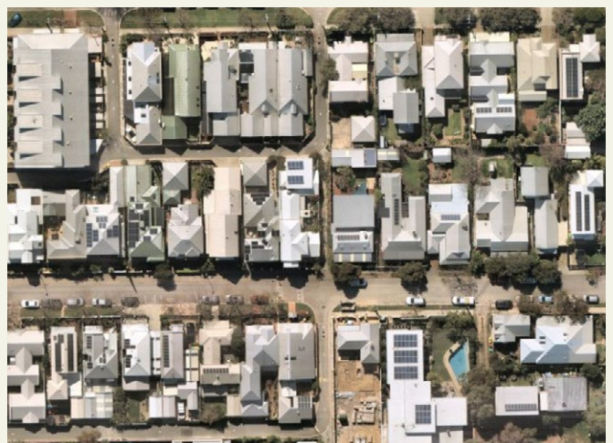
Lighter roofs reduce heat transfer
