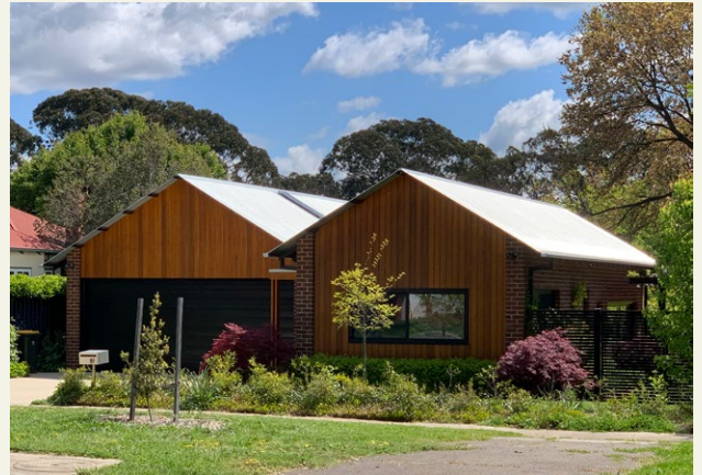
Example of a stained timber façade
