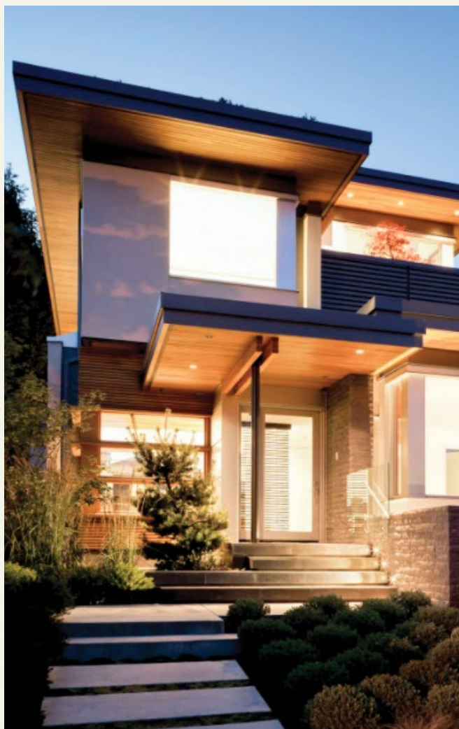
A post and beam supporting a partial cantilever style porch entry is open and welcoming from the streetscape.
