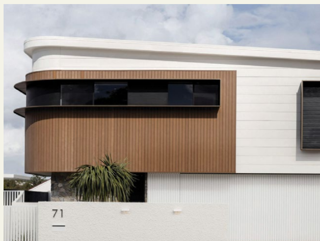
Example showing sunhoods to windows.
