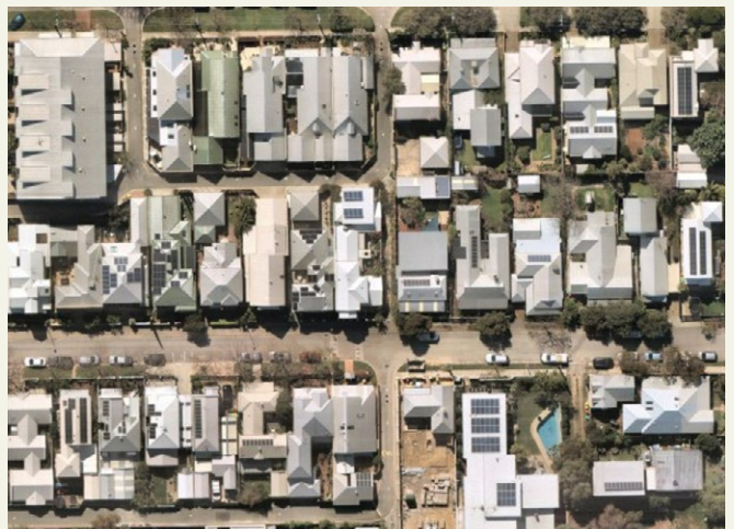
Lighter roofs reduce heat transfer
