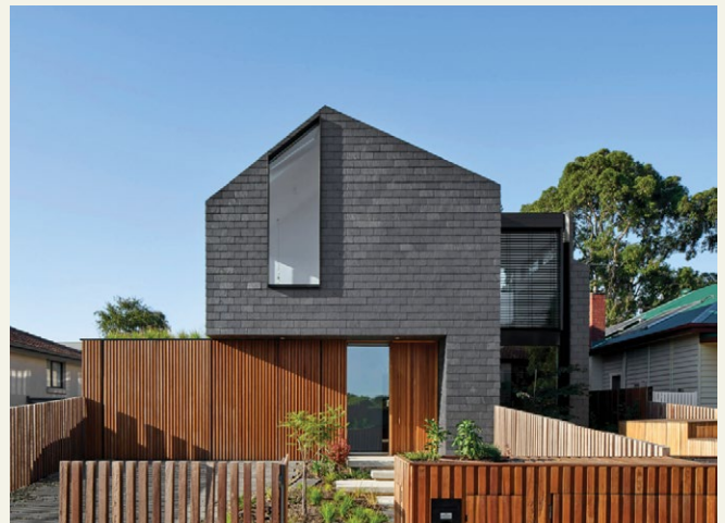
Example of integrated timber tilt up garage door and vertical timber cladding
