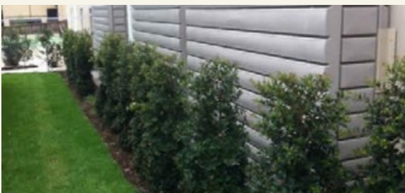
Narrow style rainwater tanks can be used where space requirements are restrictive
