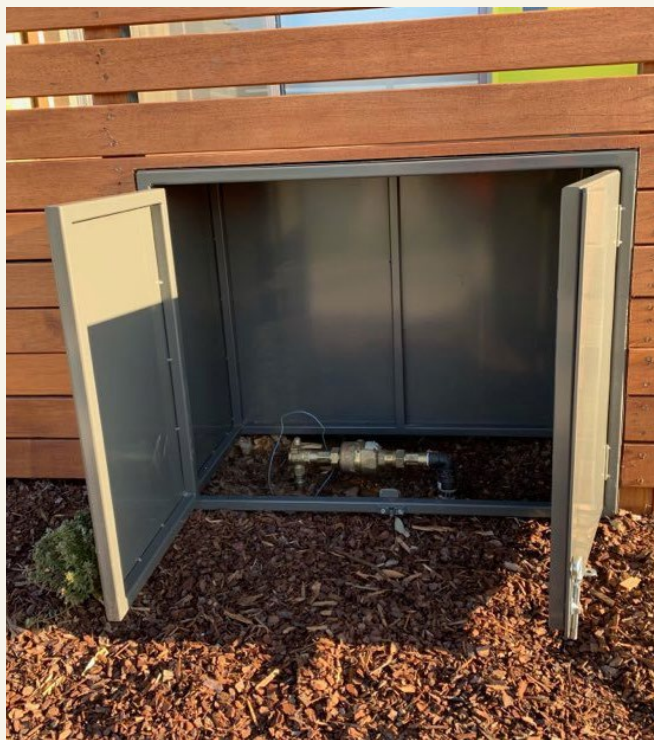
Integrated water meter details within courtyard walls
