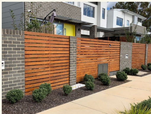
Clear entries behind courtyard walls
