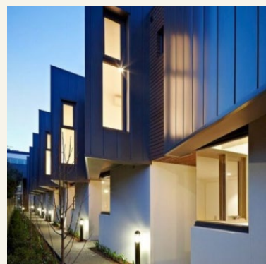
Clearly articulated facades add value and character to the streetscape
