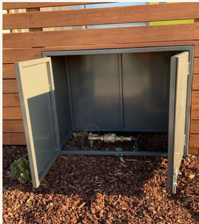
Integrated water meter details within courtyard walls
