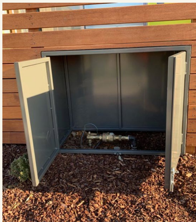
Integrated water meter details within courtyard walls
