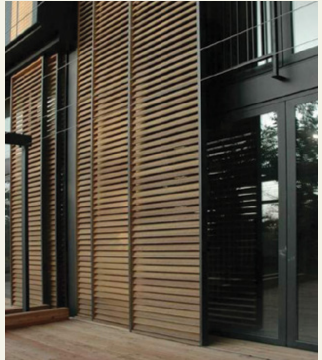
External screens to shade western façades.
