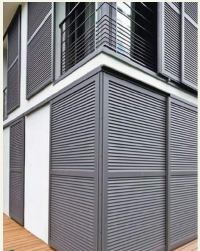
Western summer sun can only be controlled through vertical sun protection. Consider operable sliding louvres or screens to living areas facing due west.
