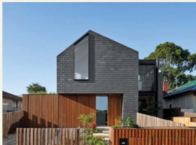
Example of integrated timber tilt up garage door and vertical timber cladding
