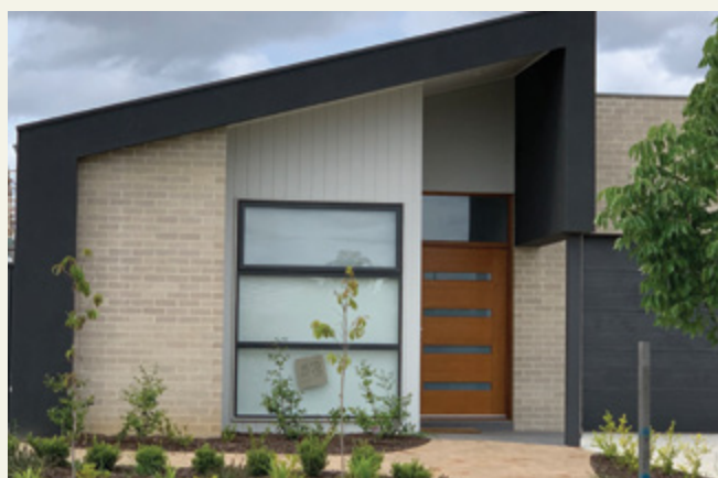
Integrated roof line and single post provides a well covered and visible entry.
