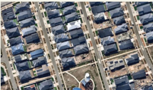
Darker roofs create excessive heat
