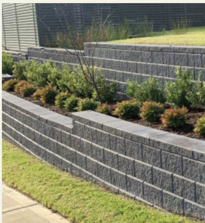
Architectural split face block with capping stone terraced to reduce a single wall height.
