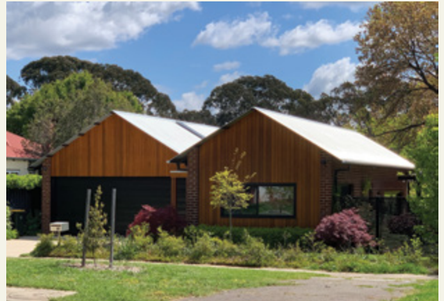
Example of a stained timber façade
