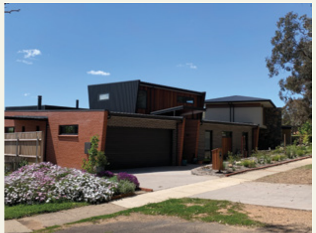
Example of face brick, cladding and stained timber to a façade
