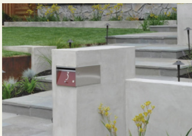
Mailbox integrated into a rendered pier and retaining wall.
