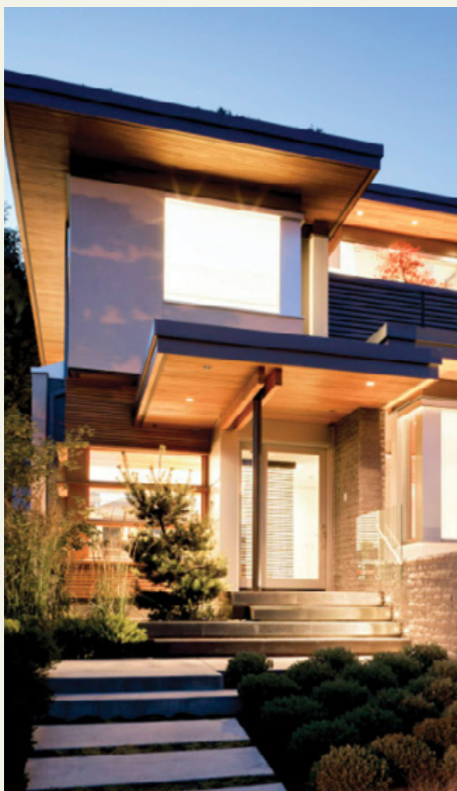
A post and beam supporting a partial cantilever style porch entry is open and welcoming from the streetscape.
