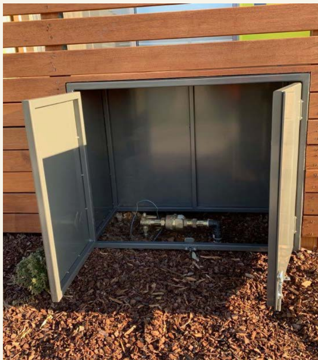
Integrated water meter details within courtyard walls
