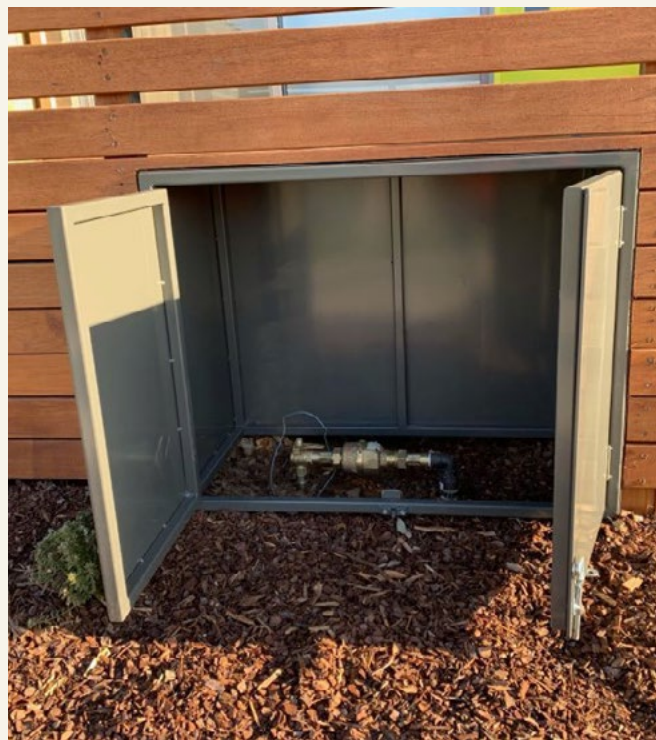
Integrated water meter details within courtyard walls
