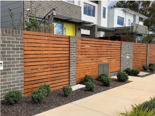
Clear entries behind courtyard walls
