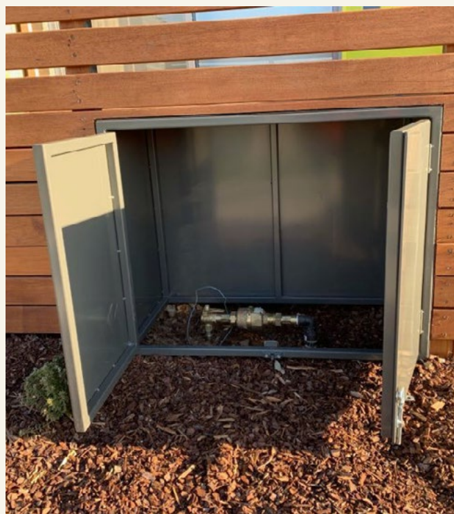
Integrated water meter details within courtyard walls
