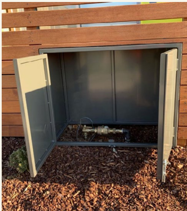
Integrated water meter details within courtyard walls
