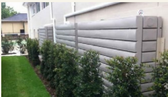
Narrow style rainwater tanks can be used where space requirements are restrictive
