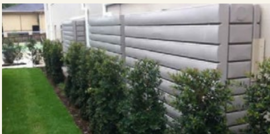
Narrow style rainwater tanks can be used where space requirements are restrictive
