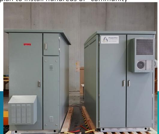
The battery consists of two main units - a battery enclosure and an inverter enclosure. The units sit on top of a 3m x 3m concrete slab and are approximately 2m tall.
