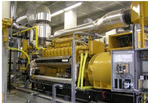
Figure 13 Installed CHP G3520C engines
