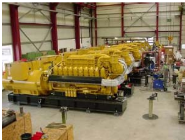
Figure 14 Installed six off CHP G3520C engines
