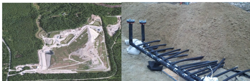
Figure 7 (Left) Aerial image of NCES Landfill; (Right) Supply and Return Line Manifold for the 10 GCHX Loops
