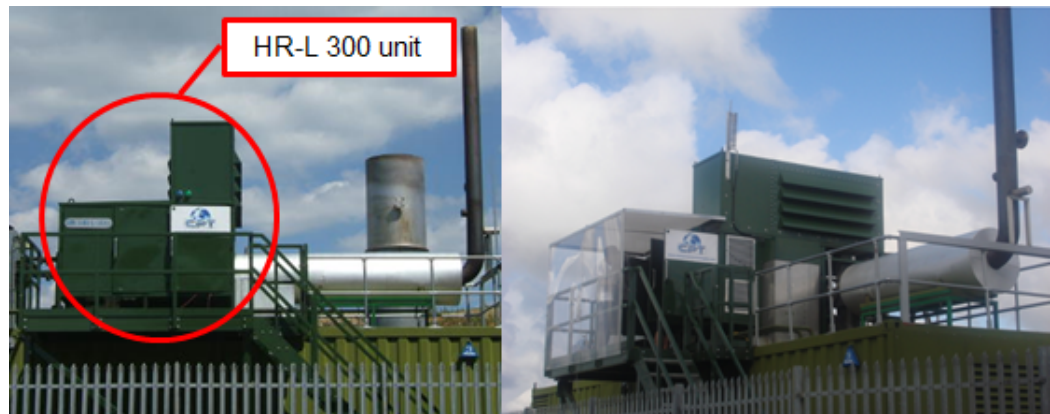
Figure 10 Installed HR-L 300 unit on the existing engine
