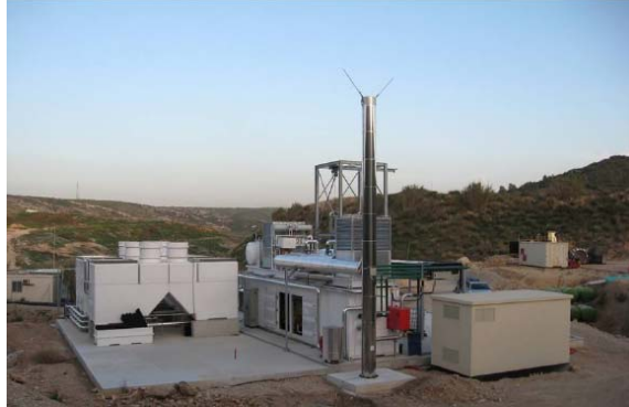
Figure 12 Installed CHP G3516A 1MW engine
