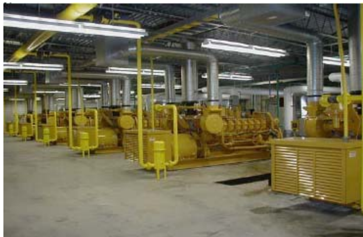
Figure 11 Landfill gas fuelled engine-generator sets
