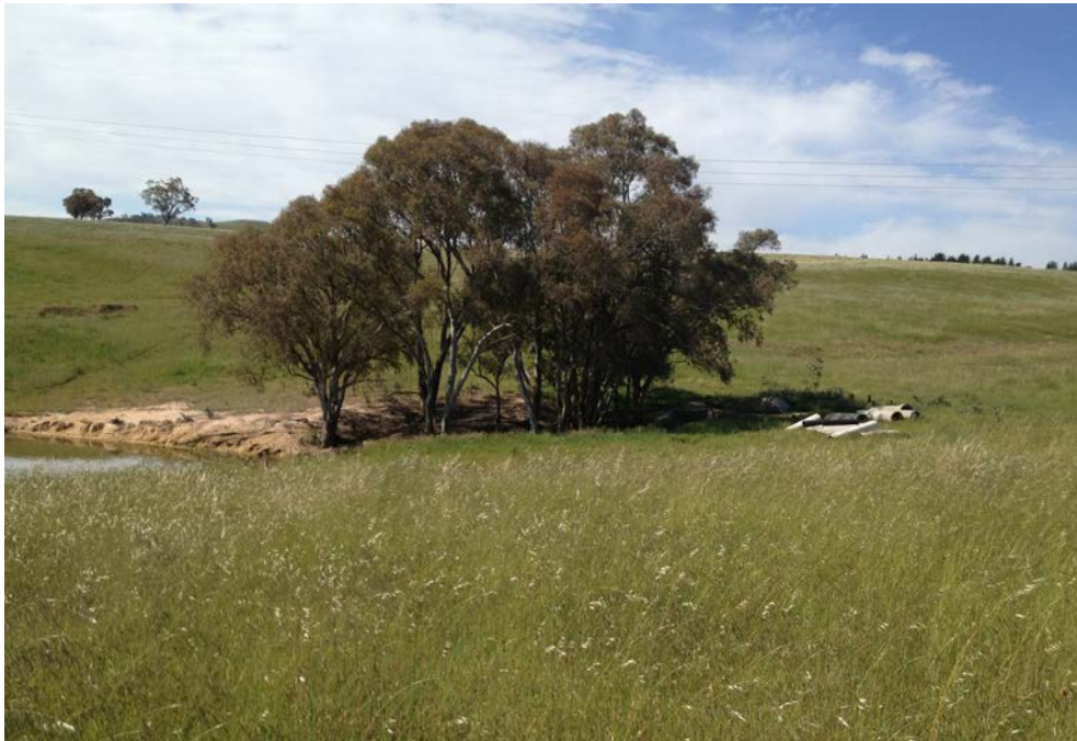
Photo N62 – Concrete pipes. Refer Drawing 4 for locality and direction
