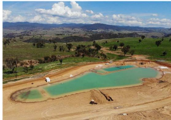
Figure 3. High Efficiency Sediment Basin (HES)
