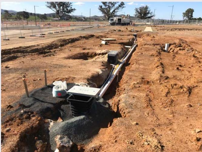
Figure 4 – Common trench service installation in Stage 1B
