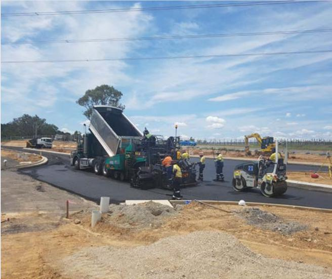
Figure 1 – Asphalt paving taking place in Stage 1A
