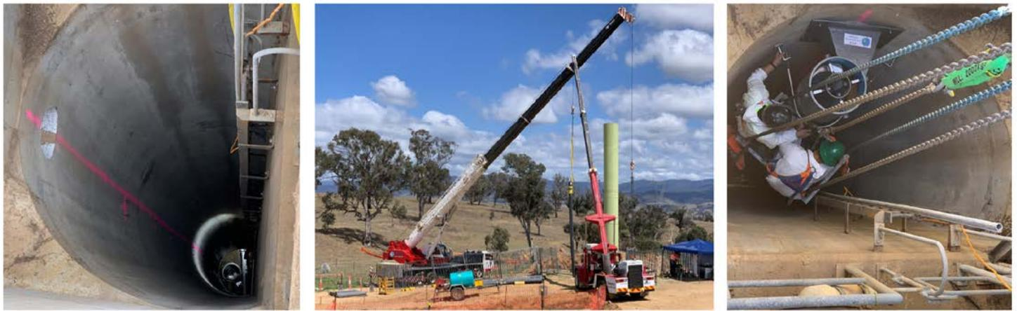
Figure 3 – (Left) View down the shaft after set out, (Middle) Dual crane setup, (Right) Vortex head installation
