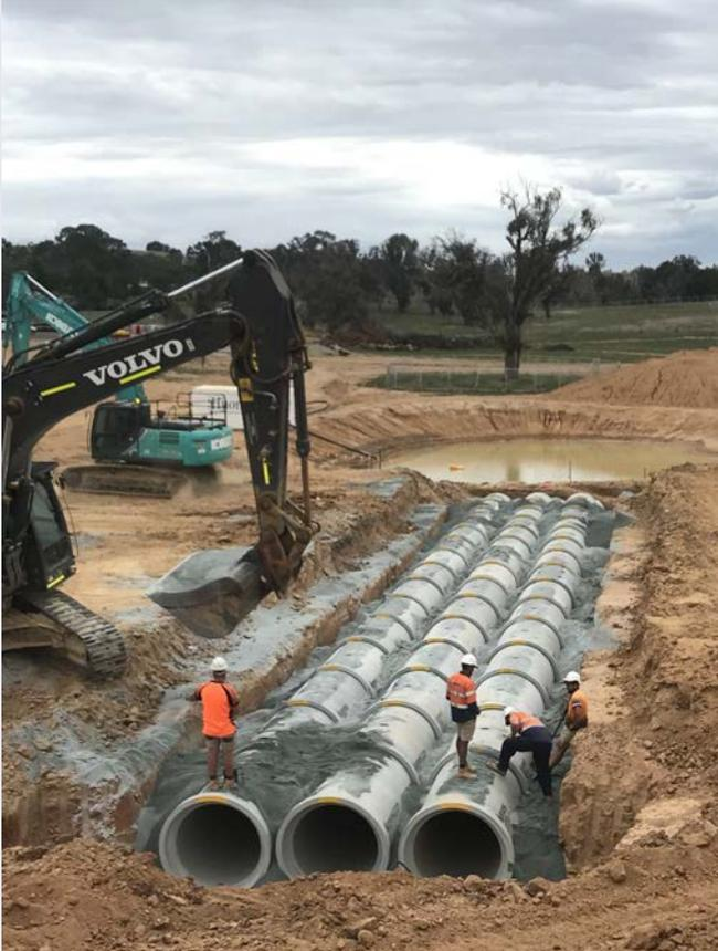
Figure 1 – Triple 1200mm Stormwater pipe installation
