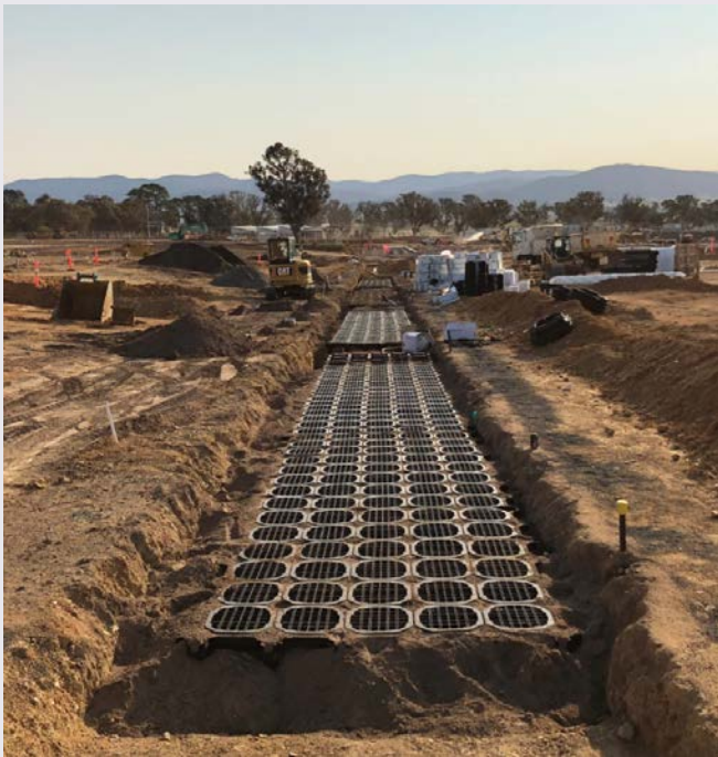
Figure 3 – Stratavault cells underneath carparking bays in the Display Village
